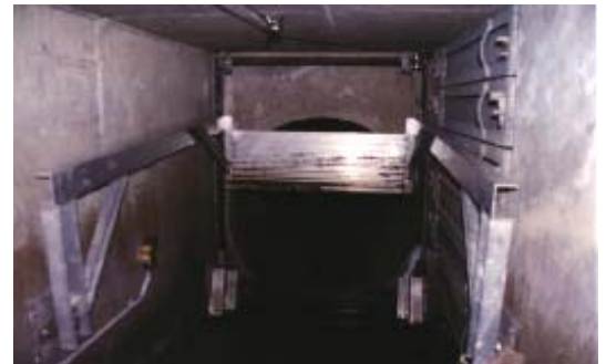
Tilting gate in open position
