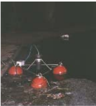
Oilspy on a basin buoy in the Sediments removal chamber
