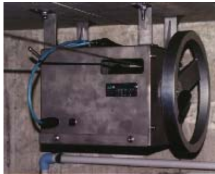
Command black box of the tilting gate
